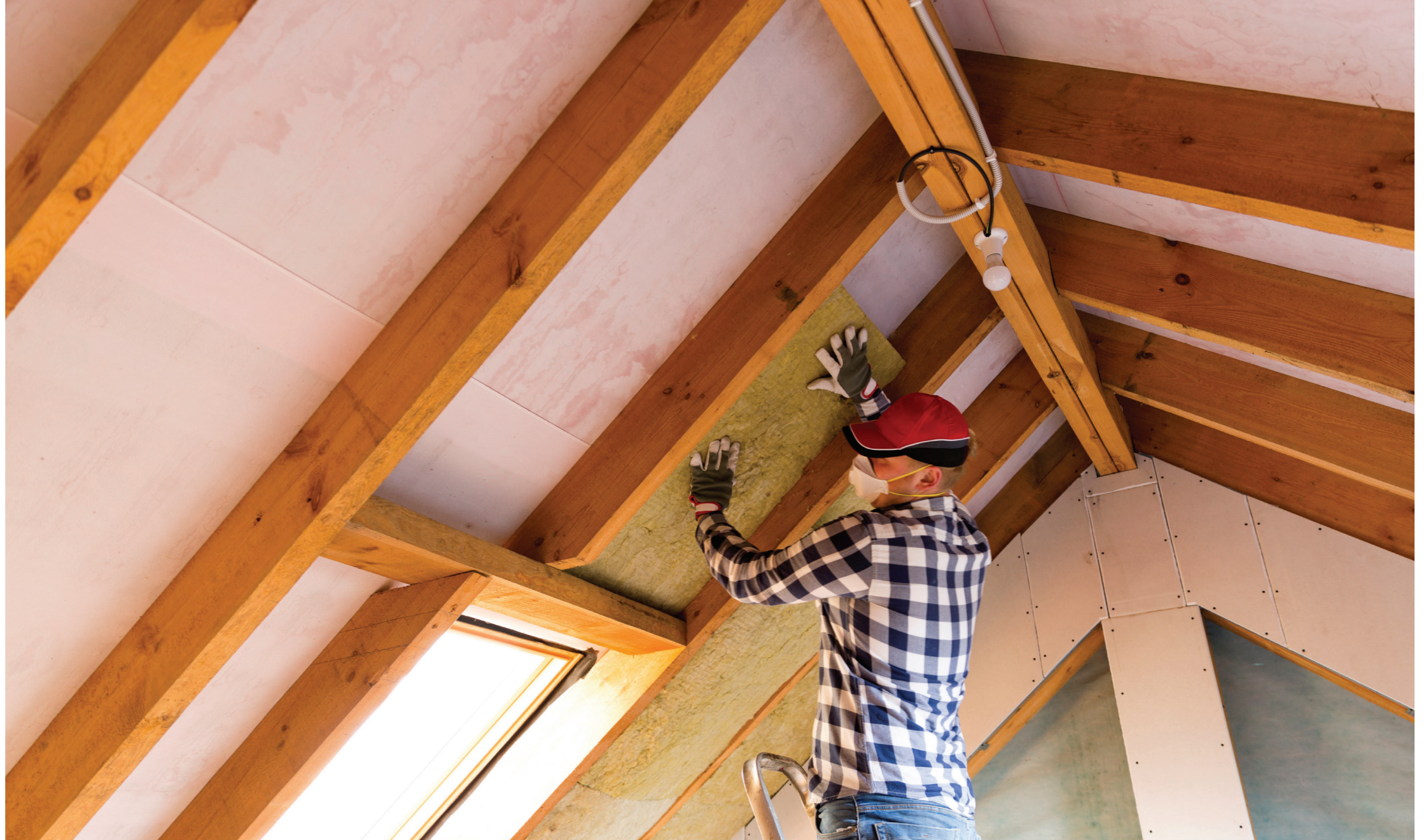
Figure 2: Installing thermal roof insulation
