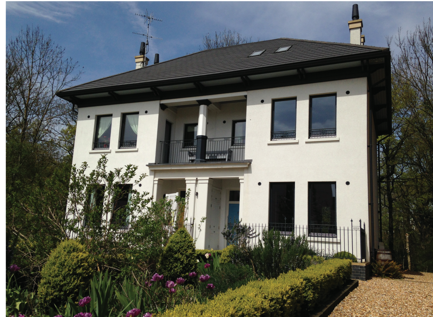
Figure 18: Experimental testing and occupancy, The Prince's Natural House, BRE, Watford
