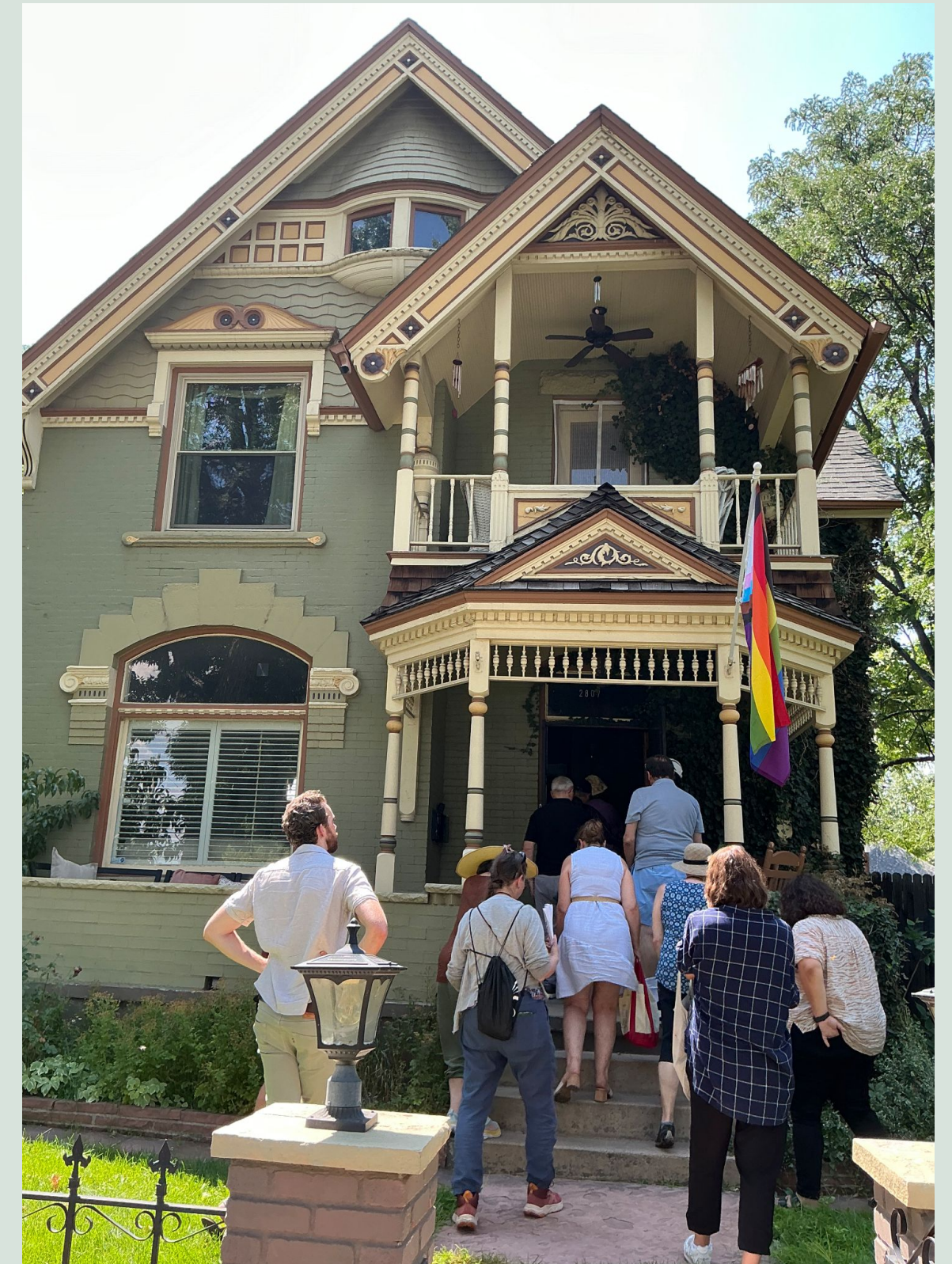
Housing cooperative, Colorado
