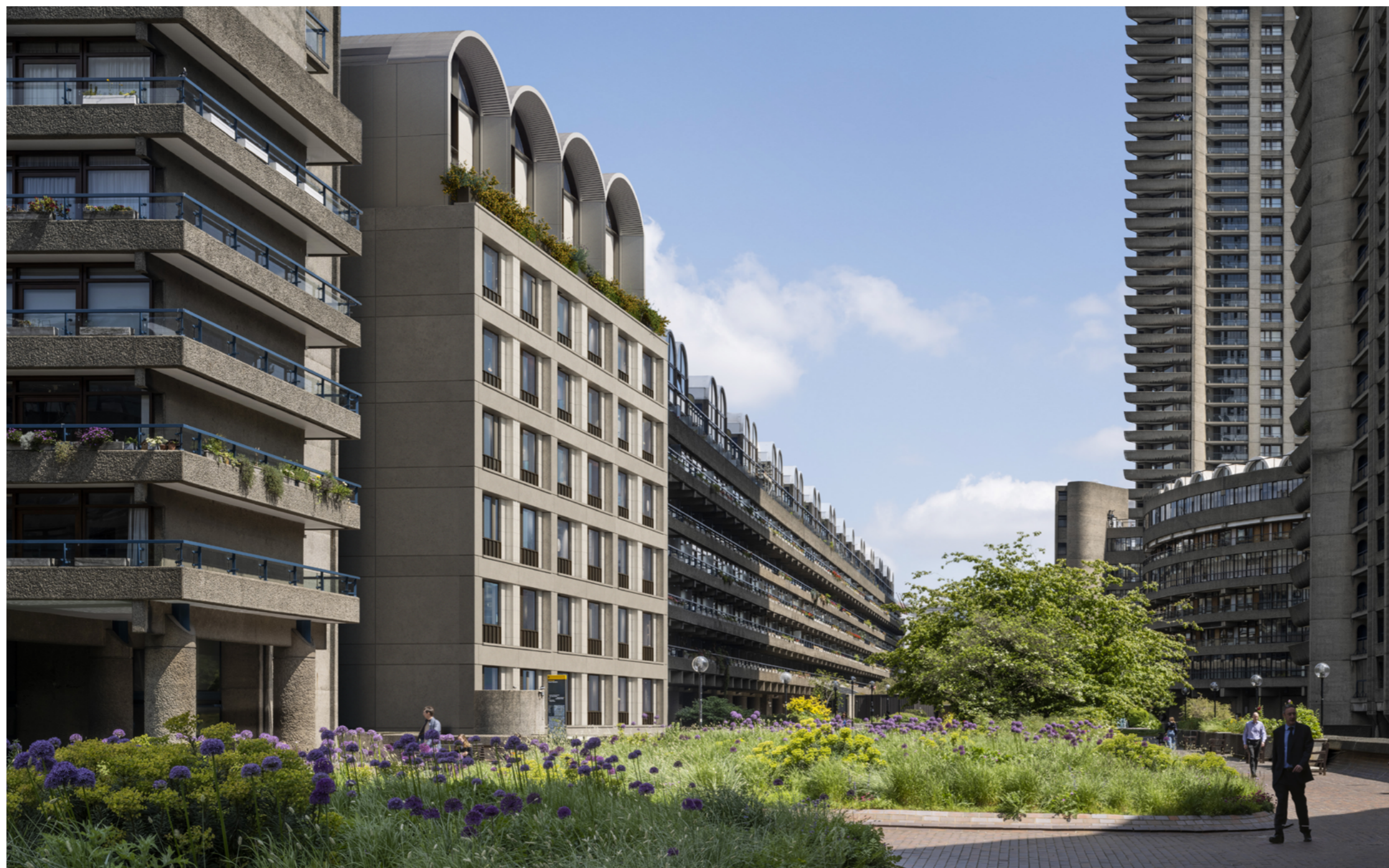
Photo credit: HUB | Bridges | AHMM
