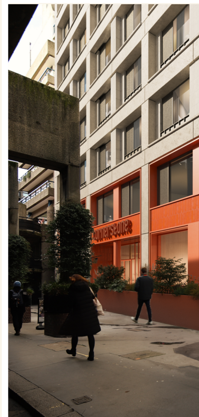
Photo credit: HUB | Bridges | AHMM
