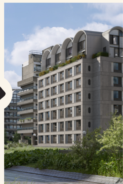
Photo credit: HUB | Bridges | AHMM
